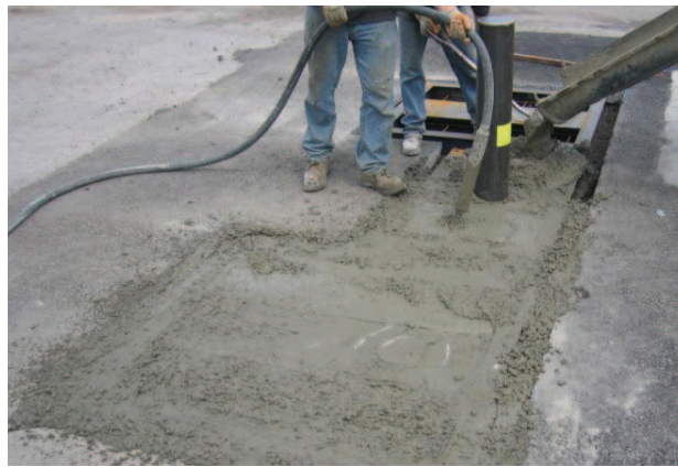
Figure 3 – Concrete poured into Foundation Installation
