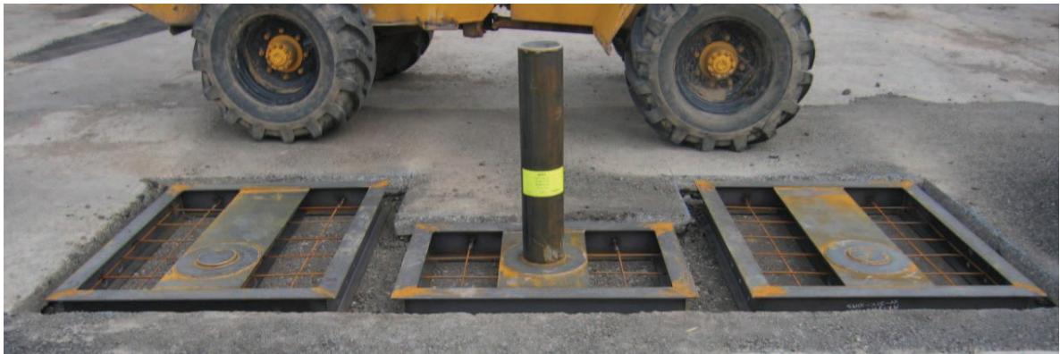
Figure 1 – Shallow Mount Units in Position
